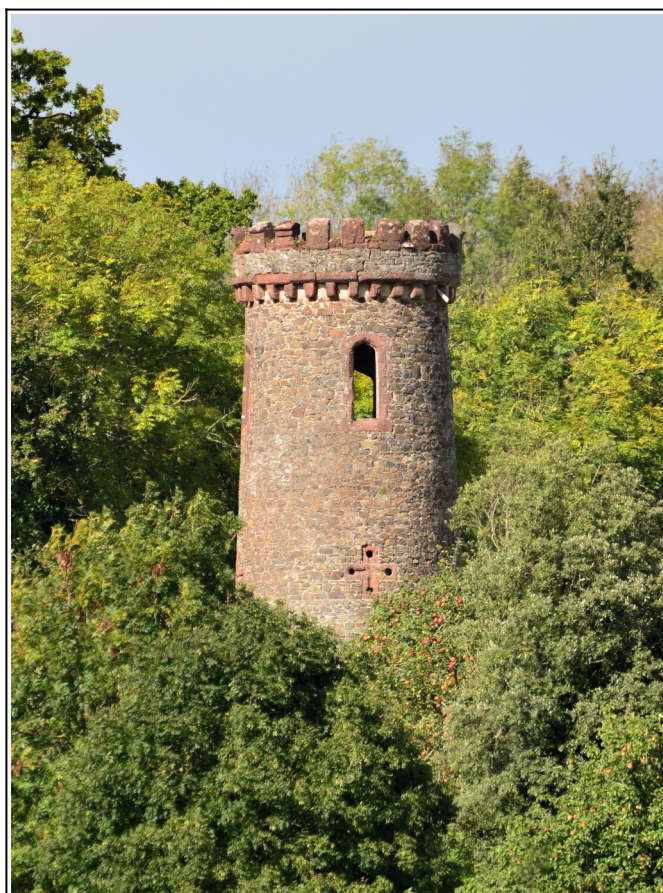
Pitt House Folly tower (as seen from the A38 overbridge near Bellamarsh Farm) © Dave Offiler
