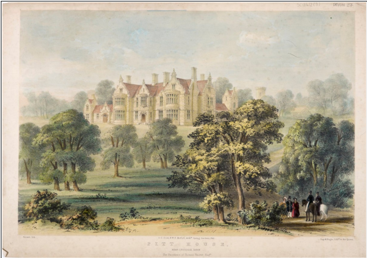
Pitt House, Chudleigh Knighton, Devon, for Thomas Painsent: perspective : 1841 Painted by Thomas James Ricauti (d. 1842) (source: RIBA Ref No RIBA83573)
